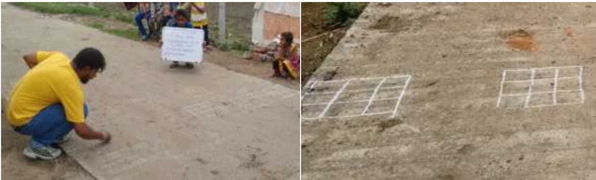
Fig.1: Grid markings on road
